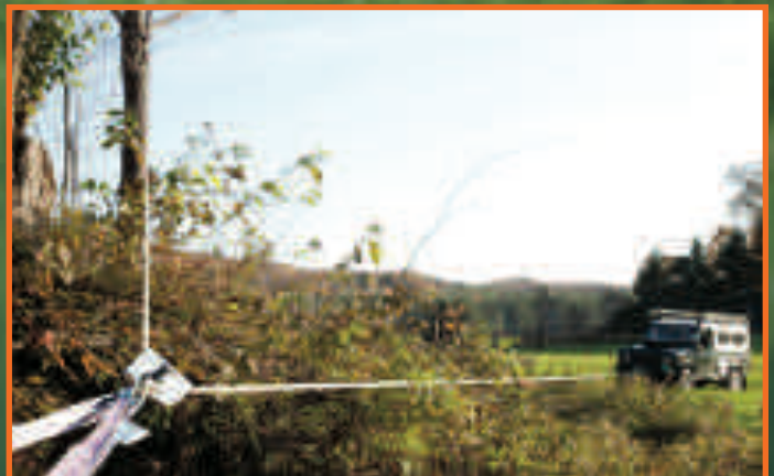
Right: The Solihull Felling System rigged before cutting.
